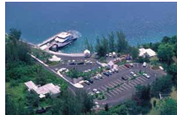
Rockaway ferry dock
